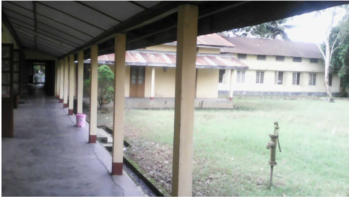
Rear view of the building
