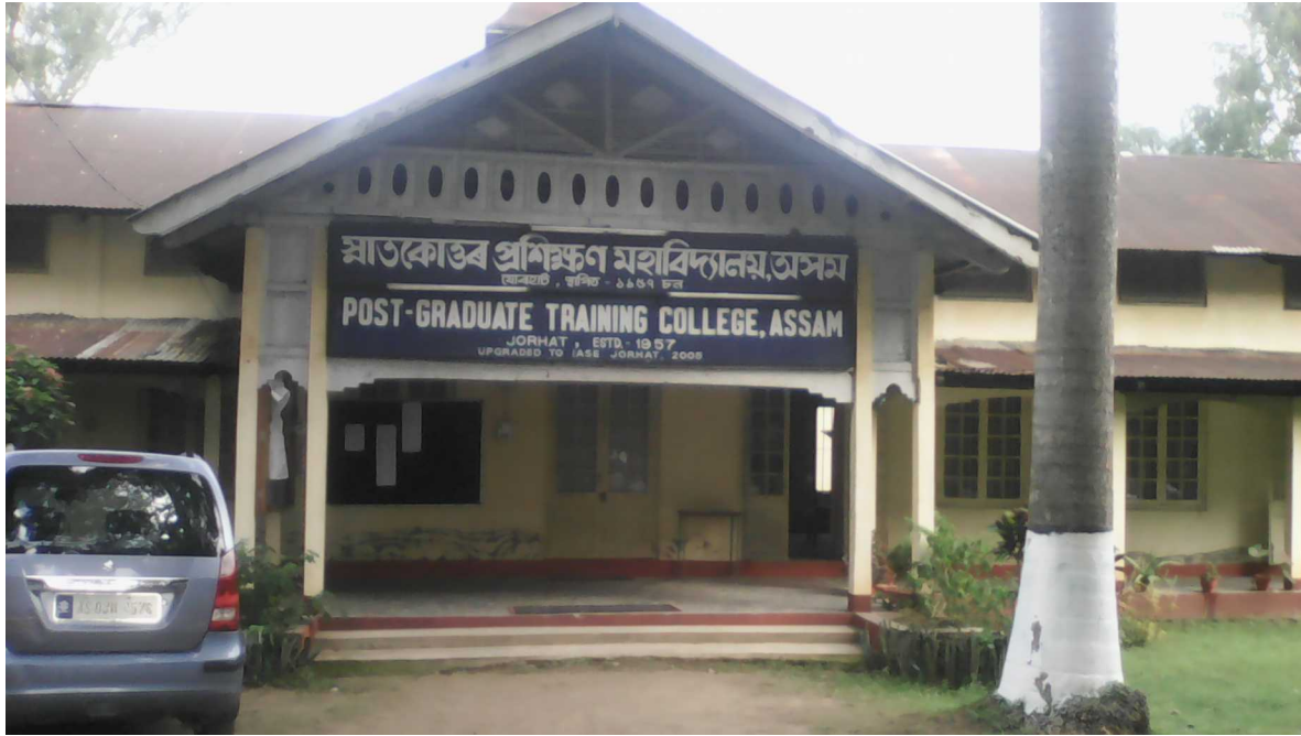
Front view of the Building
